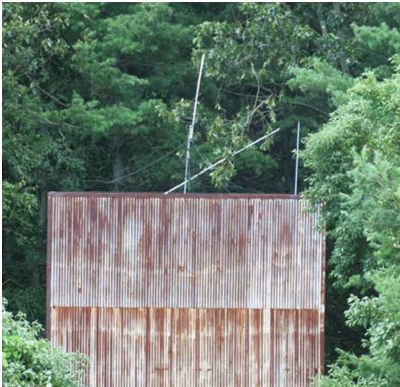
Close up of our antenna damage.
